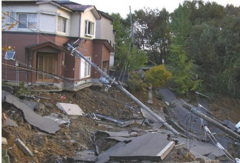
Fig. 1. Utility poles damaged by landslide.
