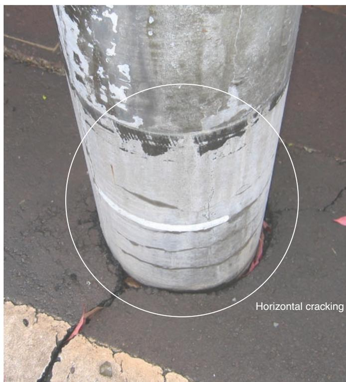
Fig. 3. Example of horizontal cracking in an urban area.
