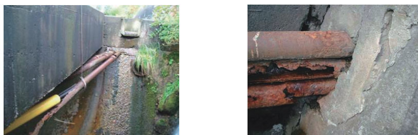
Fig. 1. Examples of corrosion (side of bridge abutment).
