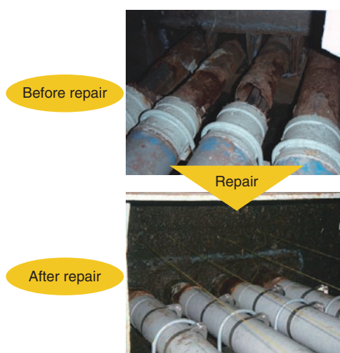
Fig. 7. Example of a repair at the side of a bridge abutment.
