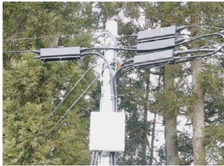
Example of use of a telecommunication cable surge protector box
