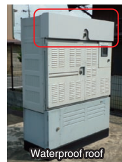
Fig. 8. Countermeasure to prevent penetration of rainwater.
