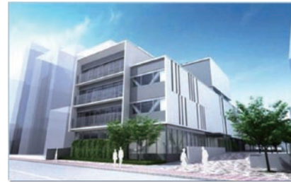
Fig. 4. NTT FACILITIES Shin-Ohashi Building.
