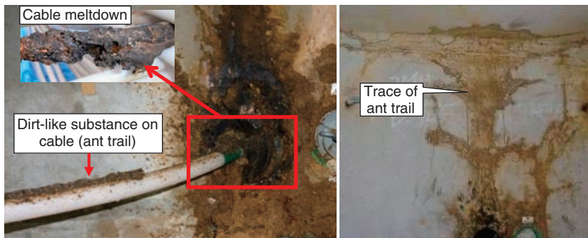
Fig. 7. Situation inside manhole.
