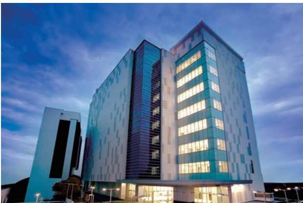
Photo 1. External view of datacenter in Jakarta.
