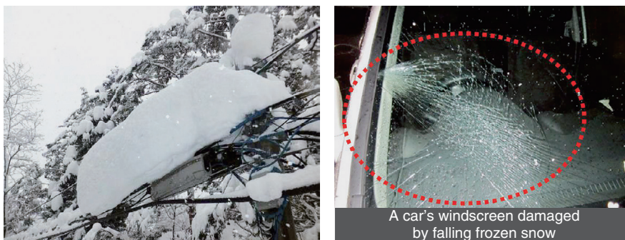
Fig. 1. Snow accretion on a closure and property damage.
