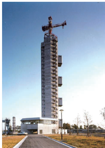
(a) Exterior view at completion (1983)
