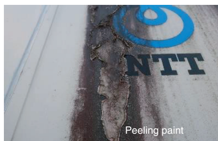
Fig. 3. Adhering substances and peeling paint on the wall.
